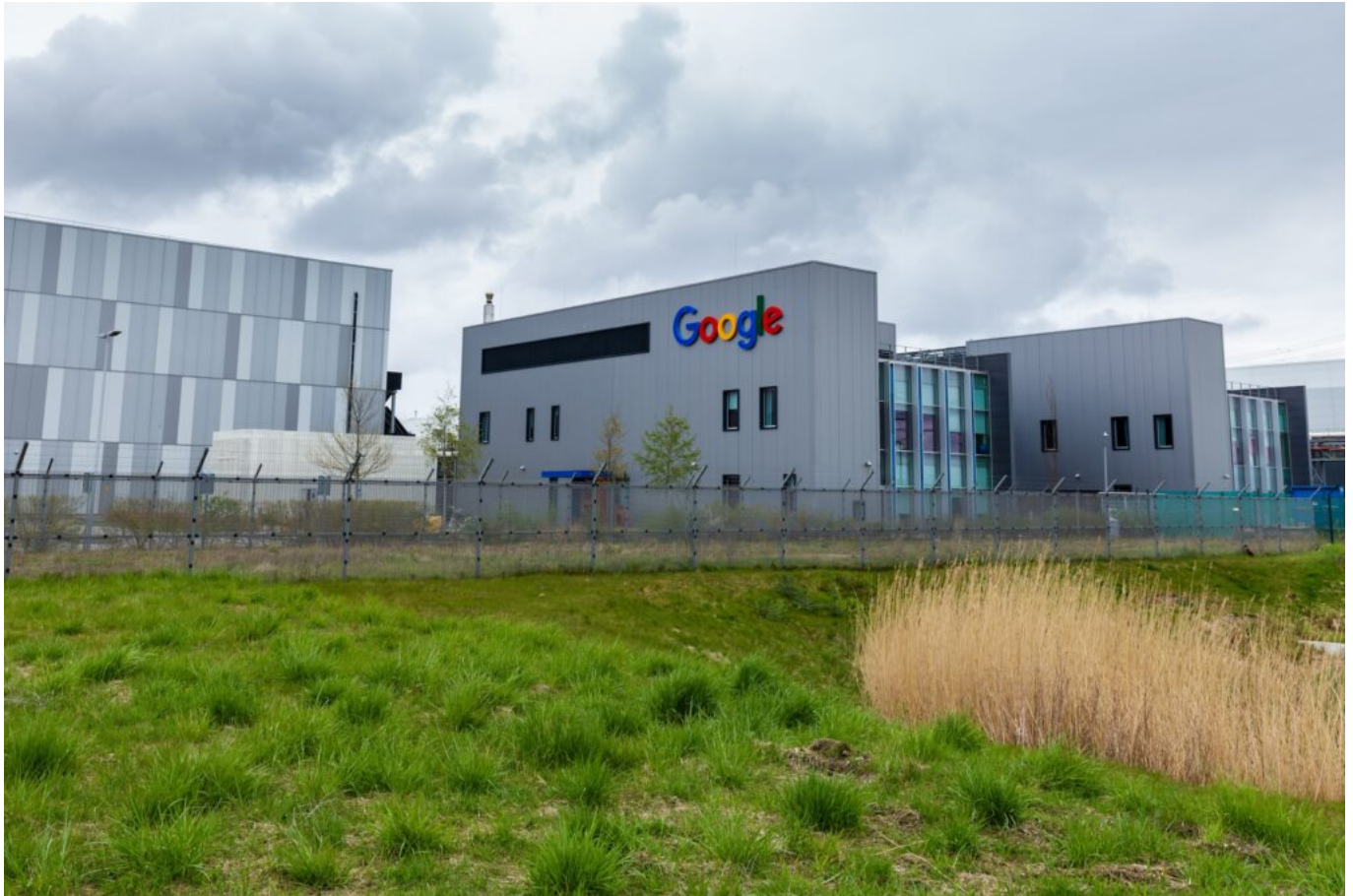
Large Google data center in the Netherlands. Photo source: Adobe Stock.
